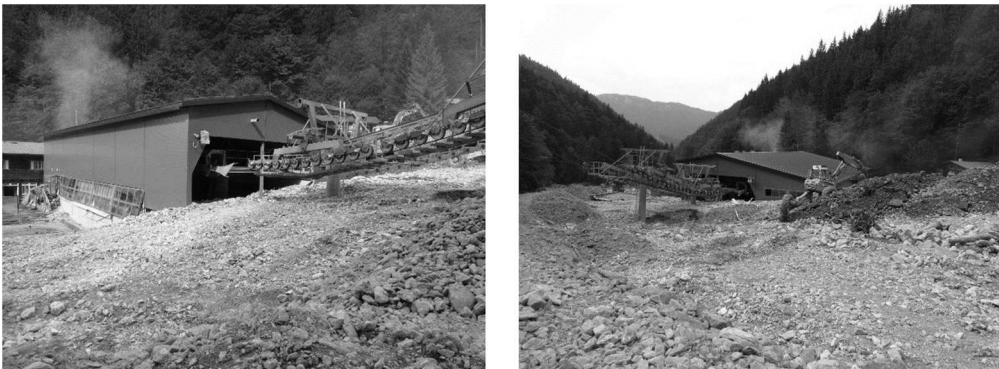
Fig. 8. Cable line terminal at the toe of the debris flow
